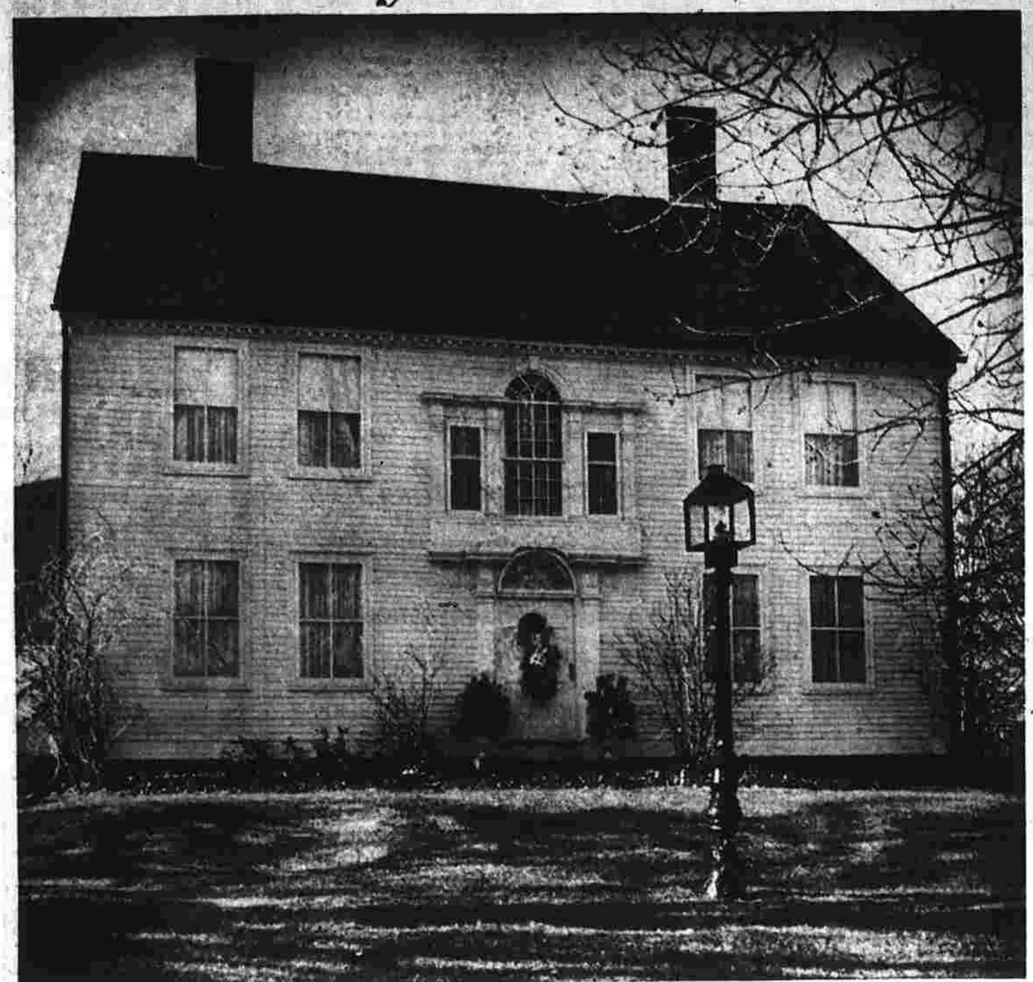
Palladian window and doorway fan distinguish the Georgian home of the E. Pierce Herricks in Bolton. . . .
